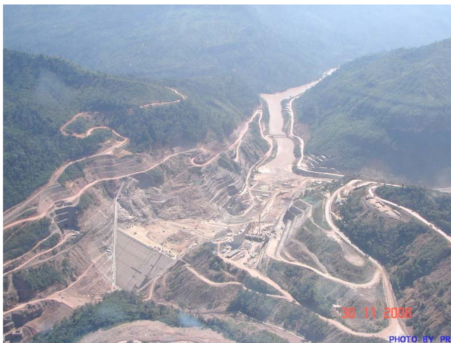
Fig. 9 Nam Ngum 2 HP Project Site under construction
